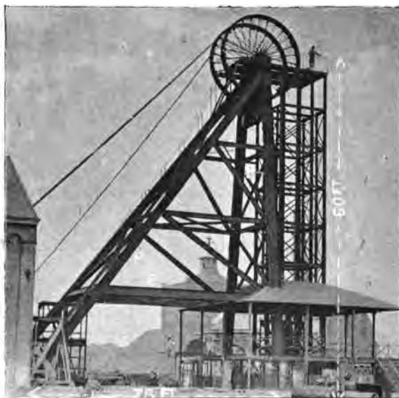
FIG. 528.—Pit-frame, plate girder (Hasard).
